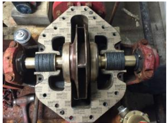
Figure 3 – Horizontal Split Case Pump Repaired
