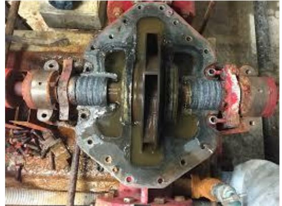
Figure 1 – Horizontal Split Case Pump Inspection
